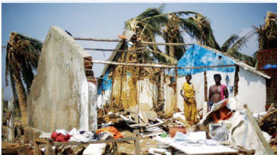
Figure 6: Showing uprooted roof and damaged house
