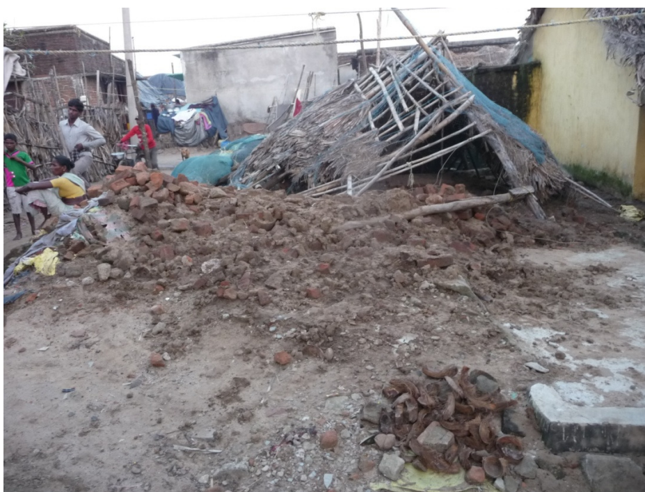
Figure 5: House completely damaged due to the Phailin Cyclone
