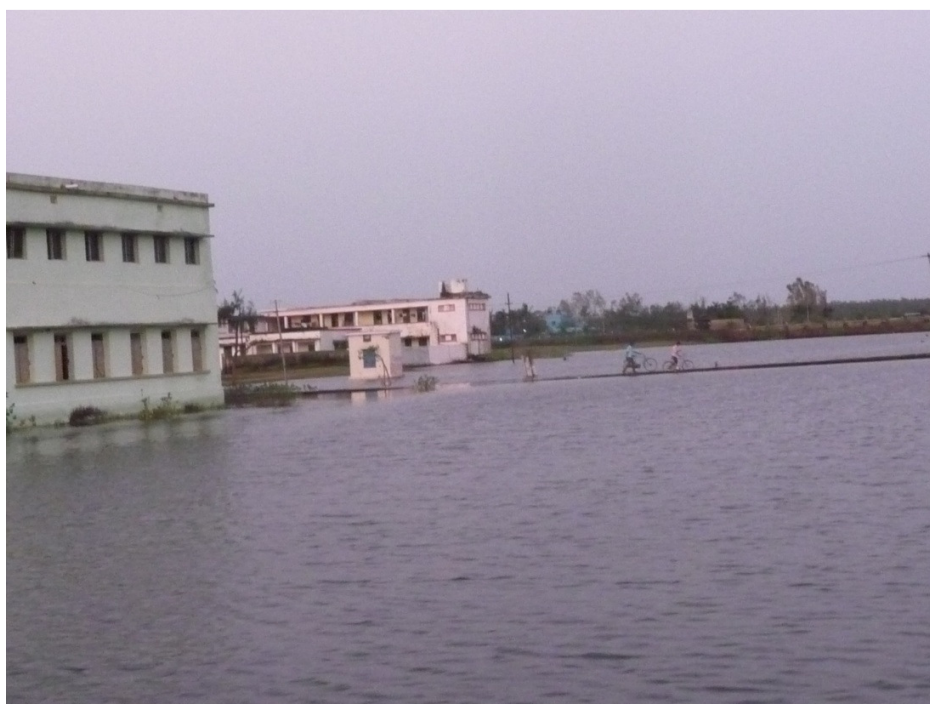
Figure 4: Showing inundated area caused by heavy rains
